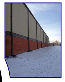
The Calgary Flames Community Arenas faced two major problems. The building was 40 years old and was in desperate need of an update. Secondly, the building's exterior stucco was cracked and either had to be waterproofed or replaced.
